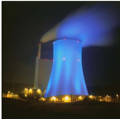
Evonik's Bexbach Power Station
