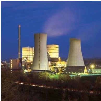
Evonik's Fenne Cogeneration Plant
