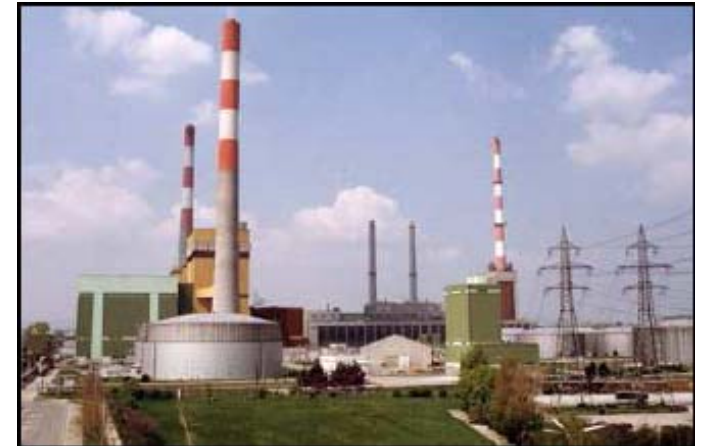
Plant Simmering (BFB)
